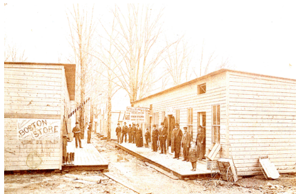
"Shanty Town." Temporary businesses located on the current village green, while the town was being rebuilt. April or May 1896.
